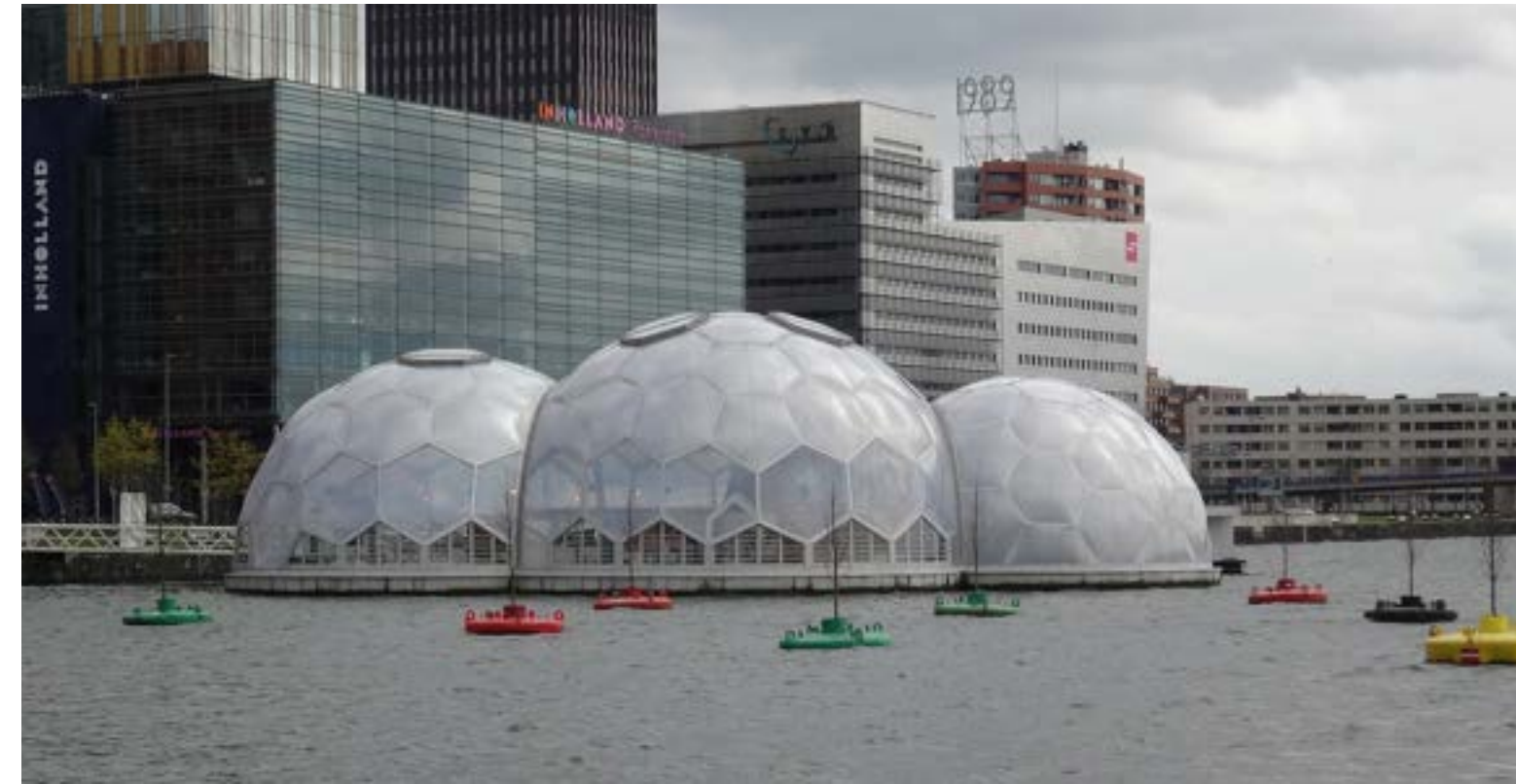
Rijnhaven Floating Pavilions, a center for demonstration and innovation in tackling climate change. Image credit by: Harry_nl, via Creative Commons.
