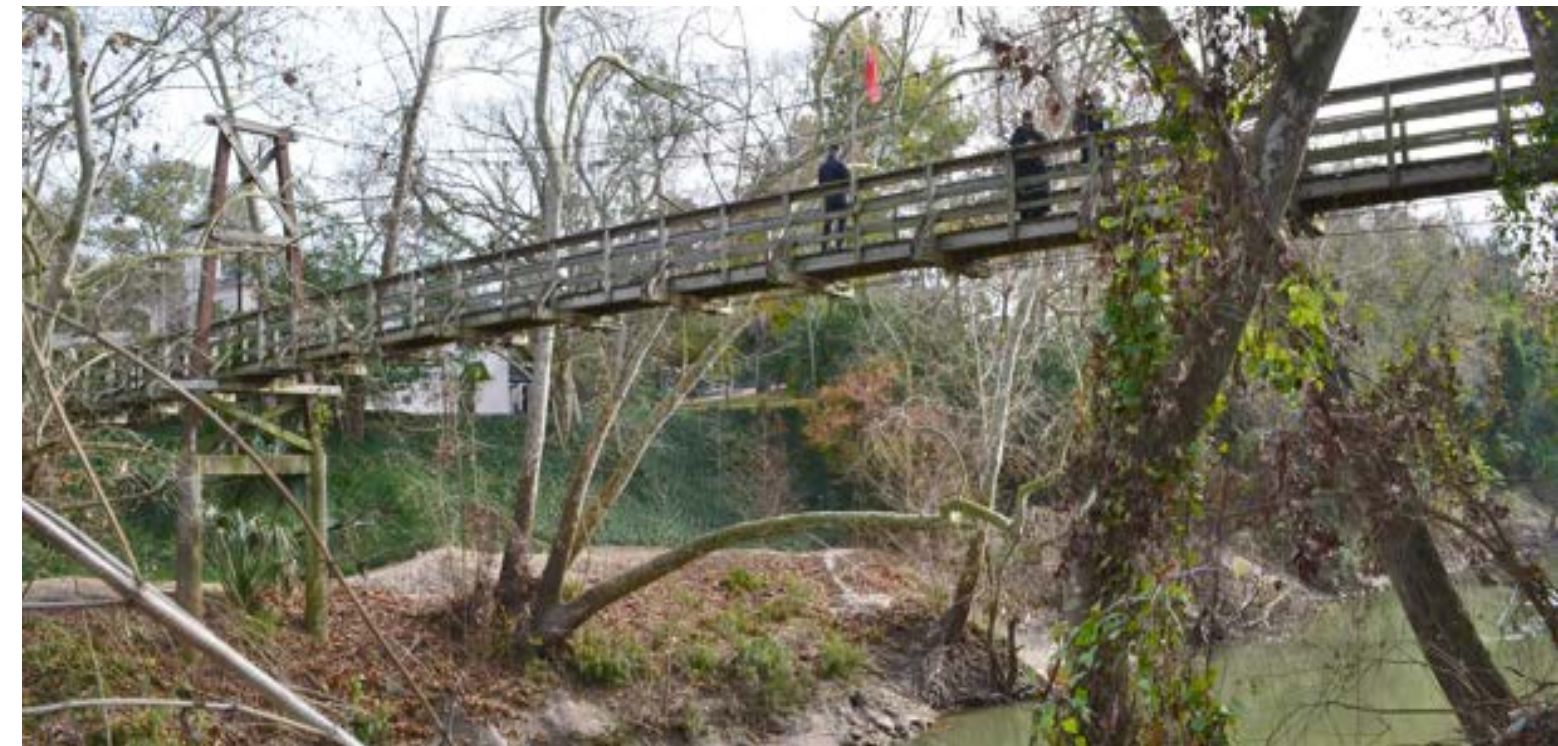
A pedestrian bridge over Buffalo Bayou was lifted above flood levels. Image credit: Patrick Feller, via Creative Commons
