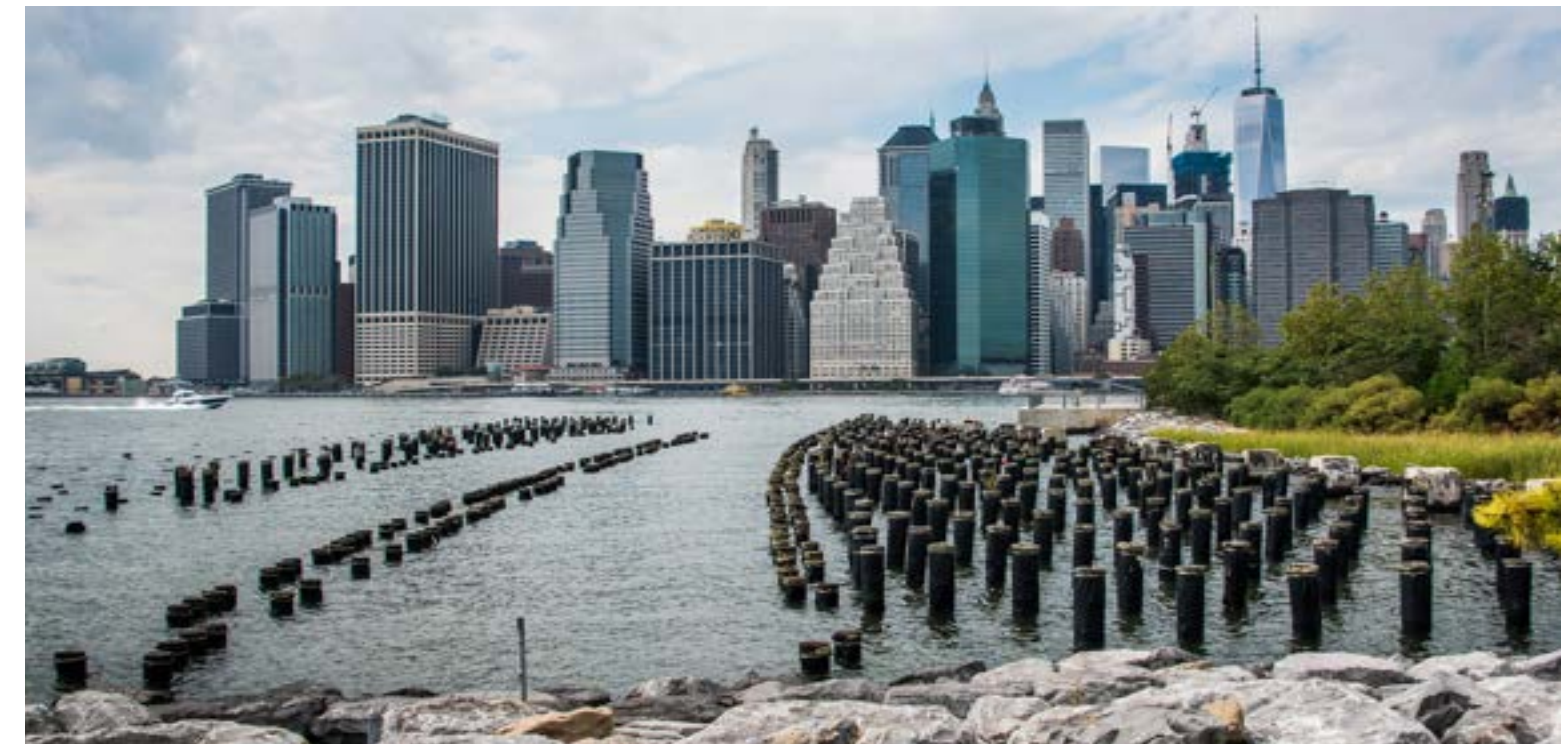
Pilings, salt marsh, and riprap stone create a porous boundary between land and water and encourage intimate interaction with the river. Image credit: Ted McGrath, via Flickr
