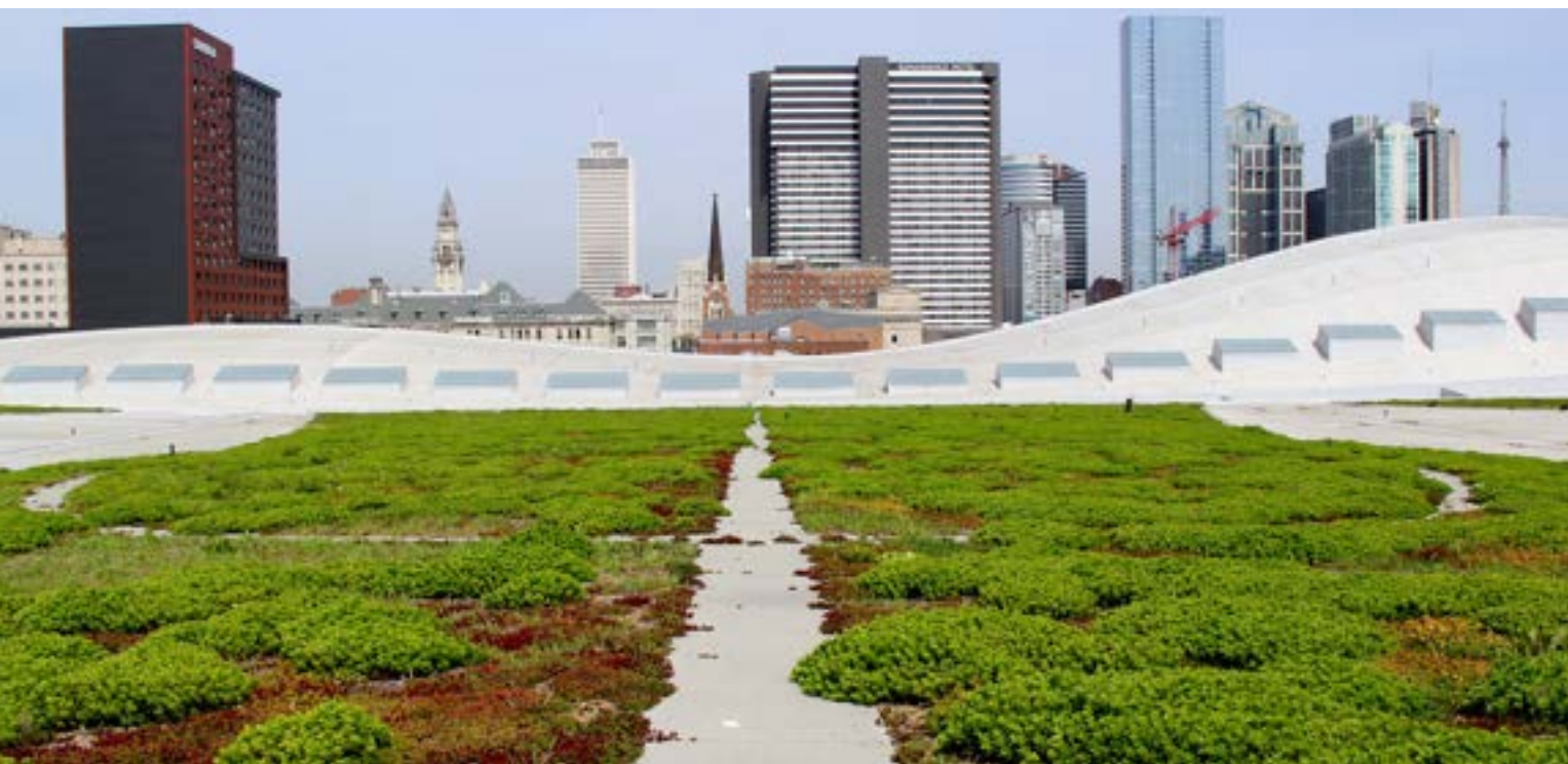
The green roof on top of the Ascend Amphitheater. Image credit: dianaconnolly101, via Flickr
